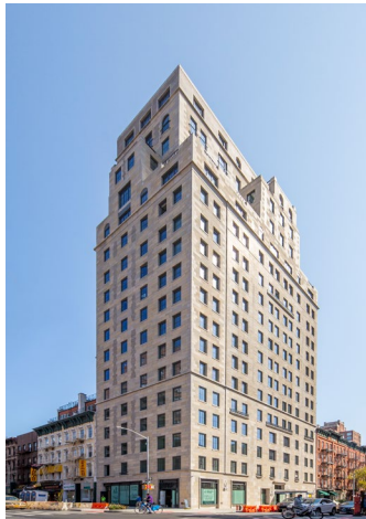
Beckford House, 301 E 81
